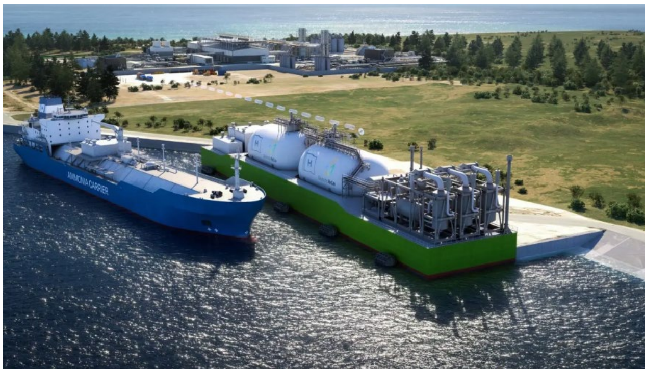
Picture: Illustration of the floating green ammonia-to-hydrogen cracker alongside an ammonia carrier.
